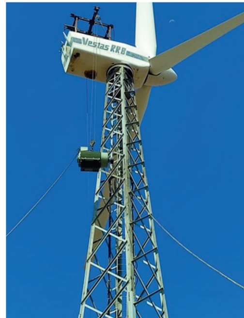
Vestas RRB 225kW Generator De-Erection
