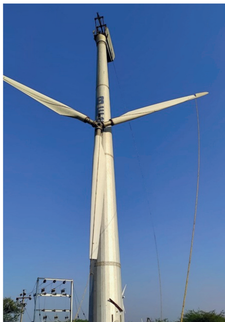
250kW NEPC Blade De-Erection
